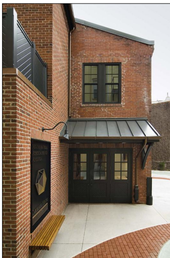
MAA Carriage House
